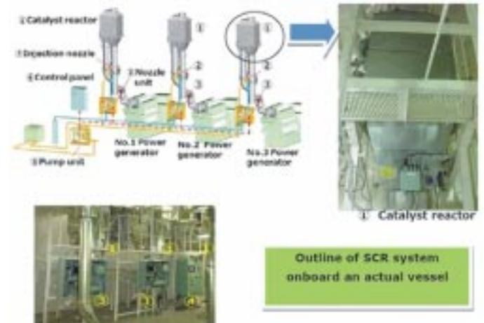
With the cooperation of Yanmar Co., Ltd. (President: Takehito Yamaoka; Headquarters: Osaka City, Osaka), we installed SCR systems on the vessel to be operational from its delivery in December 2013. Since then, the systems have been operated for more than 1,000 hours of testing each.
