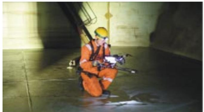
assessment and class certification. This type of inspection is usually conducted by rope access technicians who are suspended on ropes to inspect the tank structure, focusing on areas of high stress such as stiffeners, brackets, bracing, webs and stringers.
