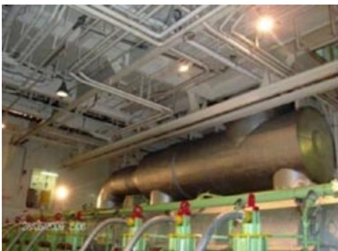
The three elements are composed of a reactive element for attenuation of lower frequencies, a resistive element-absorptive silencer to tackle with higher frequencies, and a combination element of both reactive and resistive elements. This set up will reduce the noise effectively without increasing the back pressure on the turbocharger by tuning the elements to match the engine over the noise range.
