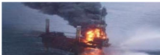
8 meters high. The collision resulted in oil and gas leakage leading to the closure of the safety valves of two production wells at the platform. The crew members were, however, unable to seal the valves completely, which resulted in continued leakage of oil and gas which ignited fire on the platform. 21 people were declared to have died during the evacuation and one worker missing in the rescue operation was presumed dead.
